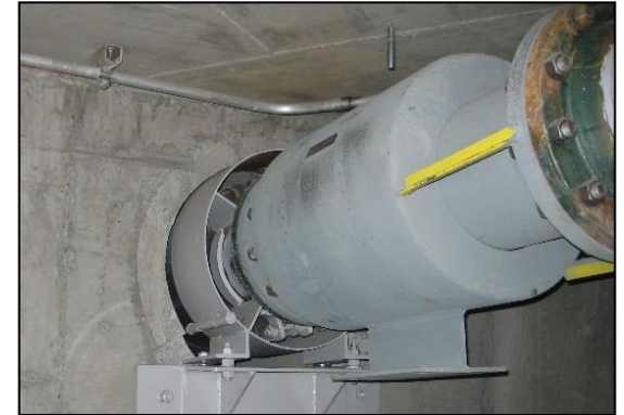
Externally Pressurized Bellows Joint
