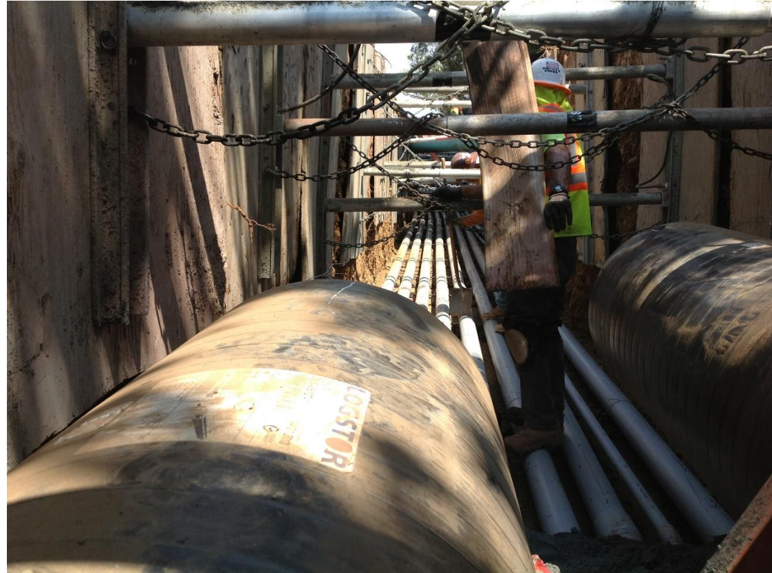
Joint Trench LTHW & High Voltage (12KV)
