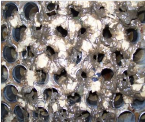
(Sept, 2008) U15 Main Condenser Tube Sheet after extended run – before cleaning, after non- MIOX treatment
