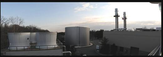
Max discharge = 10,000T at 24 °F ΔT 32 / 56°F CHWS/R = smaller, low cost, 2.7 Mgal tank Low CHWS temp = more capacity in DC network
