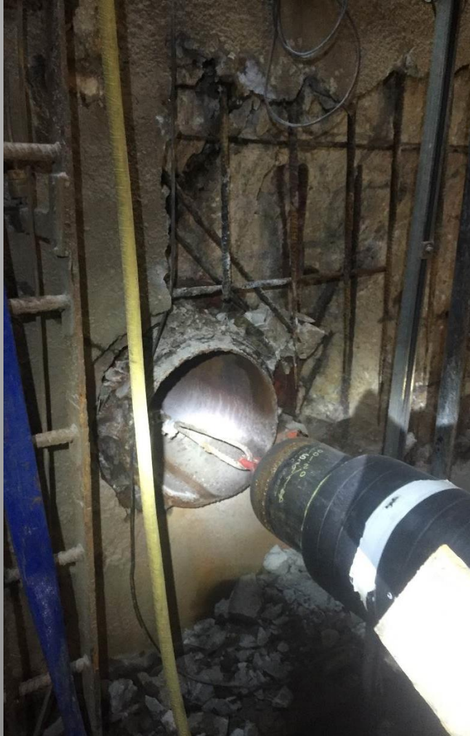
Cable pulling 10" pipe into existing 20" pipe
