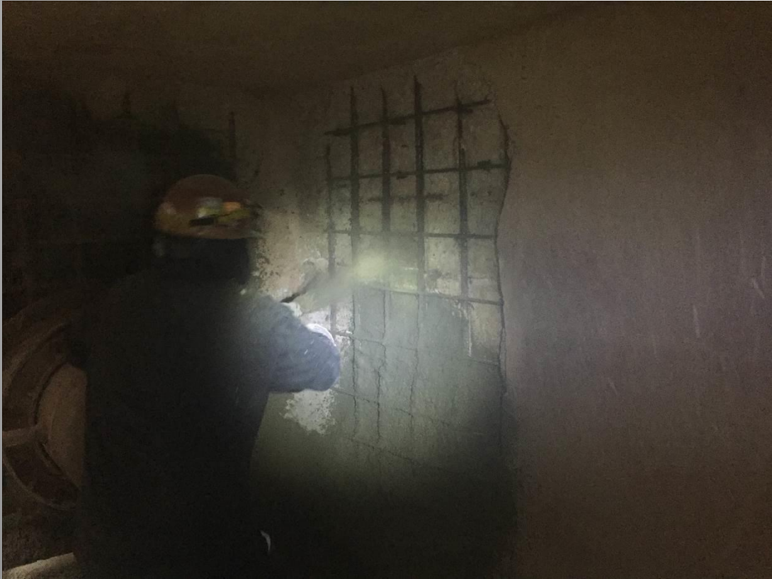
Shotcrete being sprayed in Manhole 5
