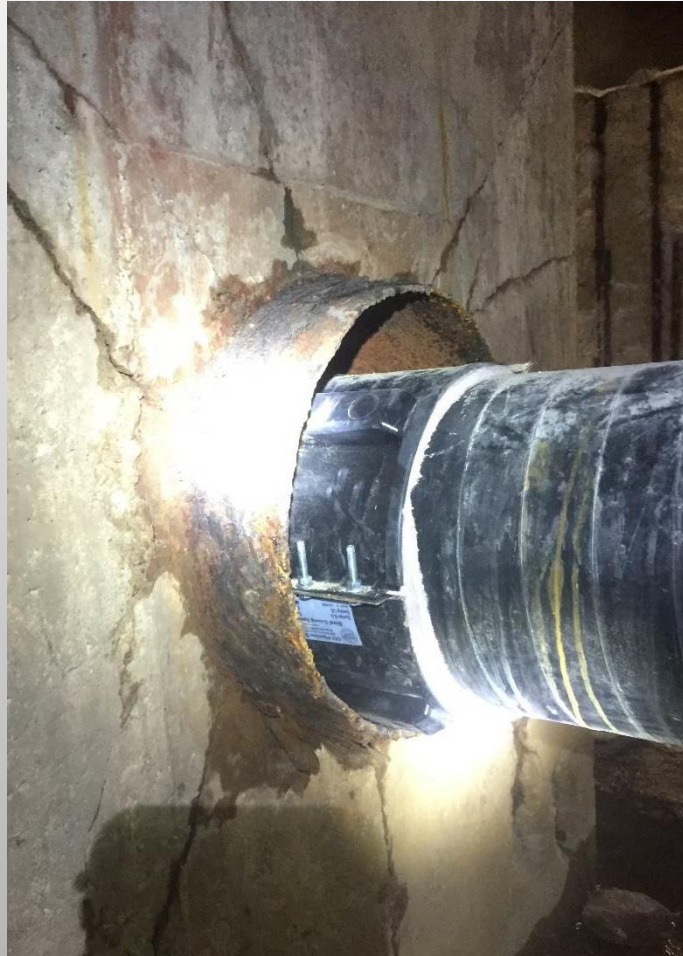
10" pipe pulled into 20" pipe between MH 25 and MH 24. Guide can be seen. 2 are installed per pipe section
