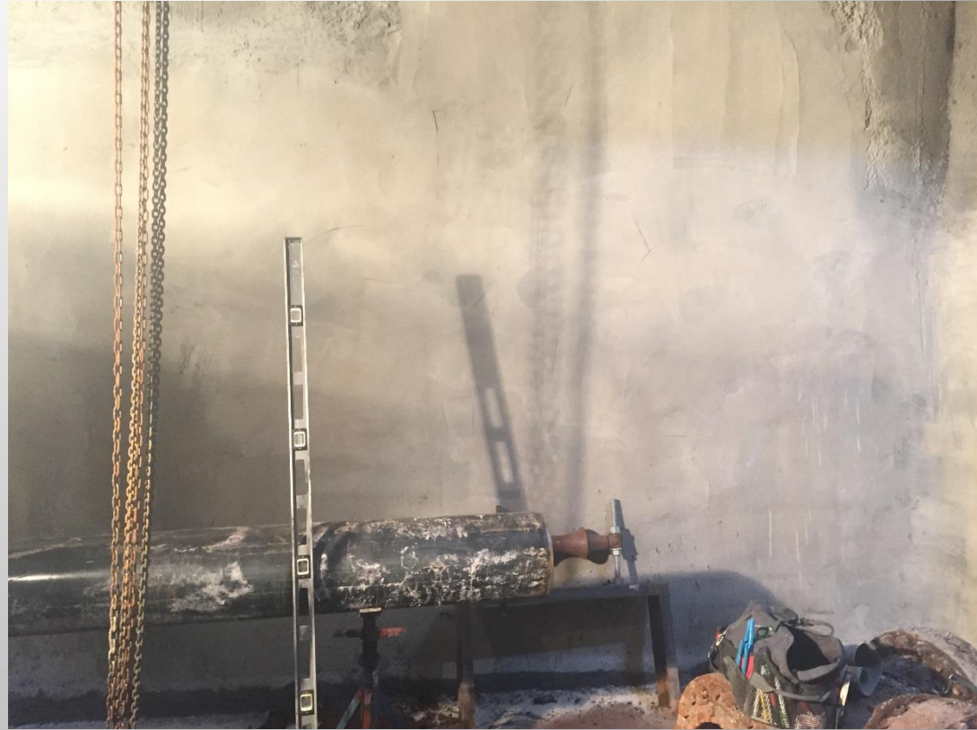
Manhole 25 wall repair Completed
