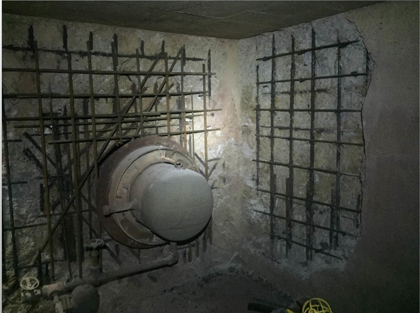
Manhole 5 wall repairs, material removed and new rebar installed
