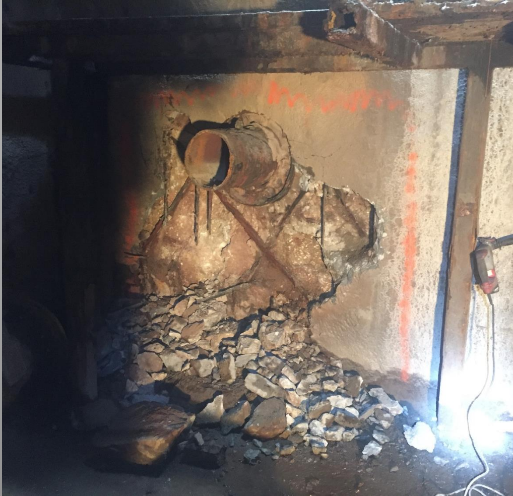
Manhole 25 wall repairs
