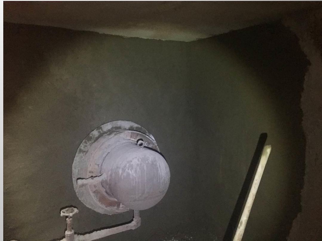
Shotcrete repair complete in Manhole 5
