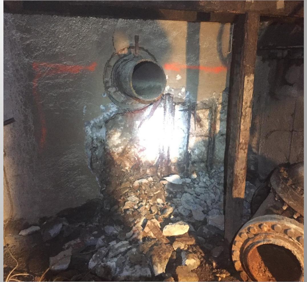
Manhole 25 wall repairs
