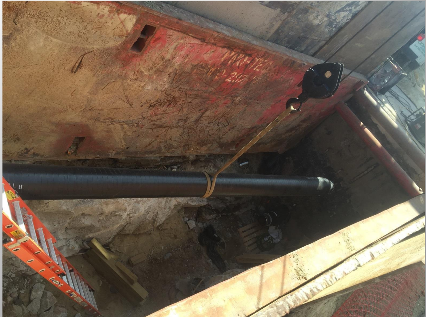
Installing Pipe in Excavation West of Manhole 5
