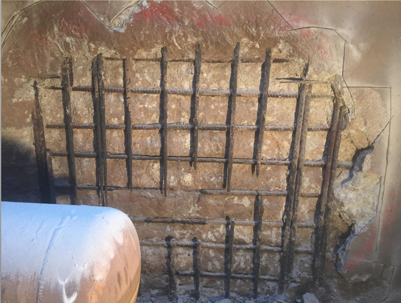
Manhole 24 wall repairs
