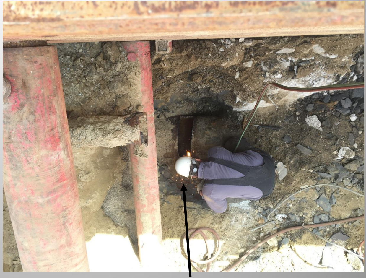
Cutting existing 20" pipe
