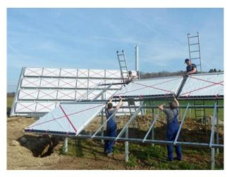
• Ground Mount pre-fabricated mounting system - 2, 3, or 4 high with 5 or 6 across
