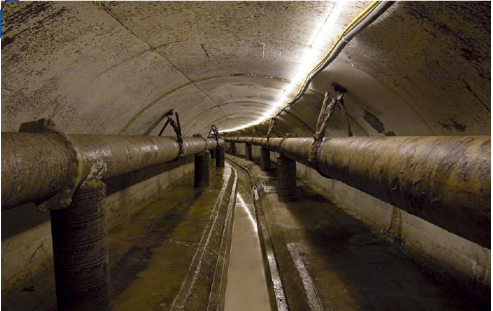
Typical Distribution Tunnel Section with Elevated Pipes
