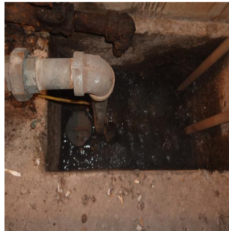
Sump Pit/Pump/Float
