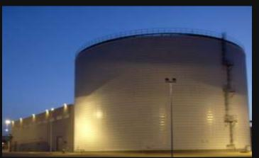
If use TIC w/ 31,000 T chillers, it nets 132 MW, at only \$435/kW! But power most valued 6 hrs/d; they used TIC w/ CHW TES, 11,000 T chlrs + 193,000 T-hrs, nets 180 MW, at only \$250/kW!! Utility uses a DC system for TIC; later, another for 40 more CTs!
