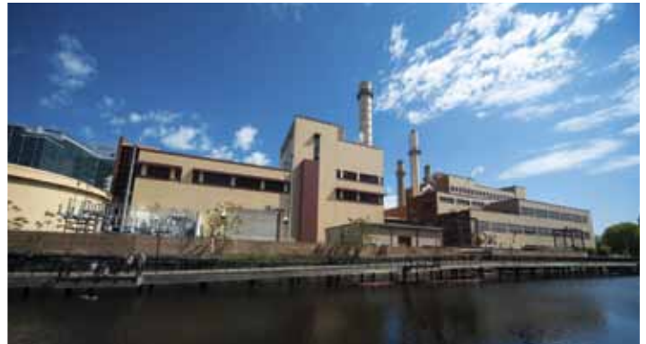
The 256 MW Kendall Cogeneration Station supplies steam to Veolia North America's district energy system serving Boston and Cambridge, Mass.
