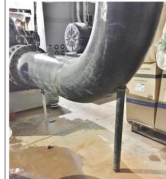
Picture to the left: The CHW pipe stanchions with vibration isolation springs are not yet installed. A temporary pipe has been welded. This installation must be completed prior to running the pumps consistently
