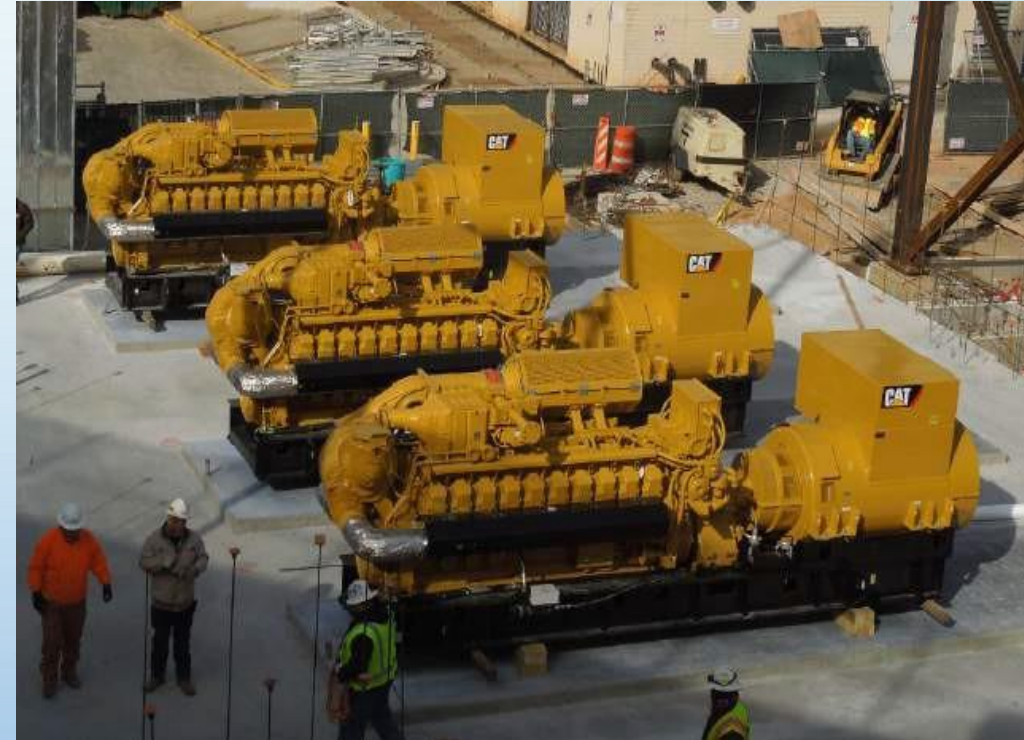
Three- 2.5 MW Caterpillar Gen-sets
