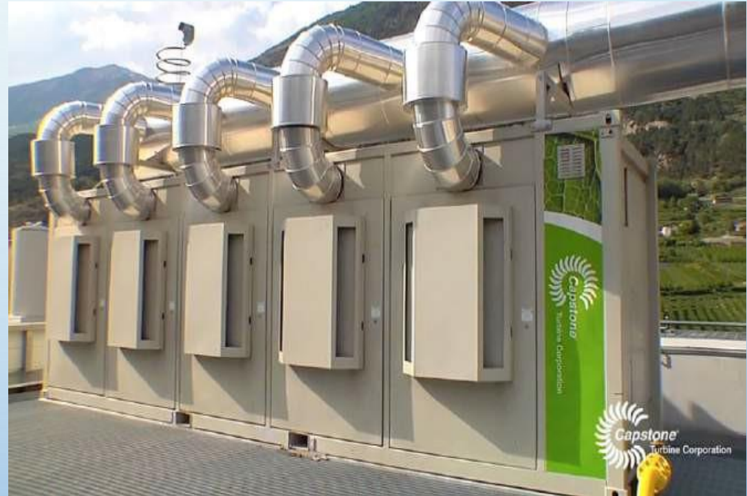
200 kW Microturbines-Courtesy of Capstone
