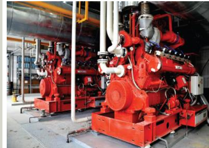
Siemens Guascor SFGLD360 natural gas reciprocating engine installed at the Grand Hotel VIDGOF CHP plant
