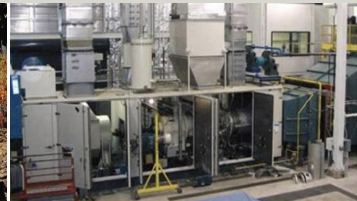
Siemens SGT-300 gas turbine installed at the UNH Cogen plant
