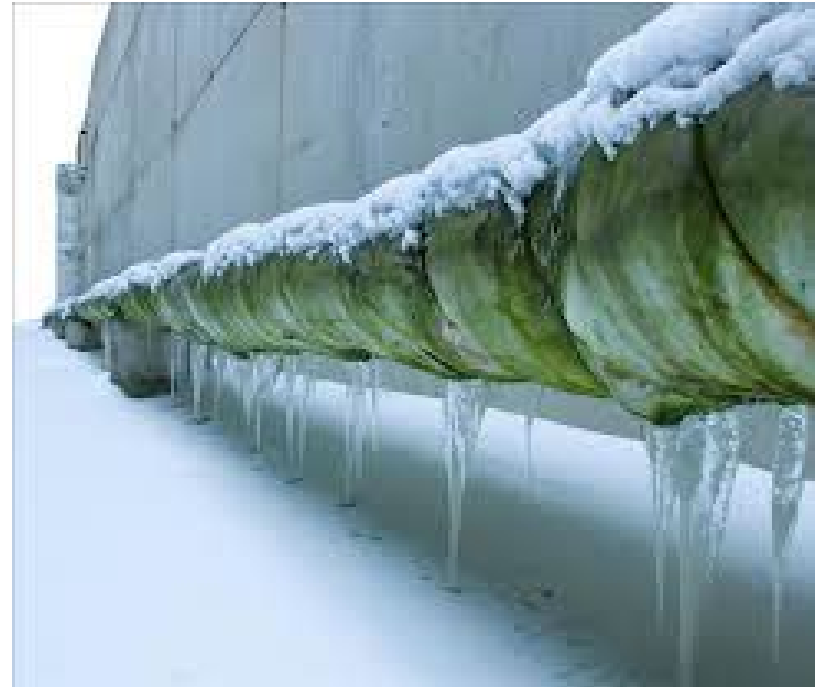
POORLY INSULATED WATER MAIN
