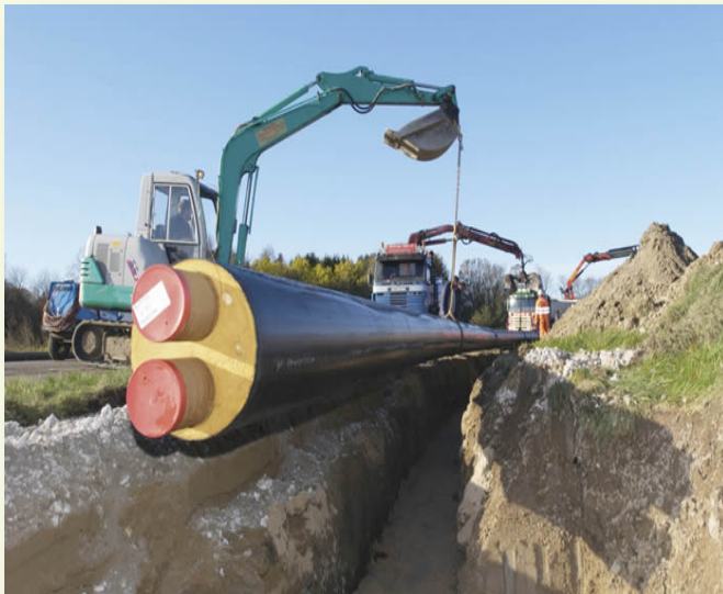
Pre-insulated piping being installed
