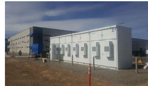
1MW/ 2.1MWh Battery Energy Storage + Islanding Switch
