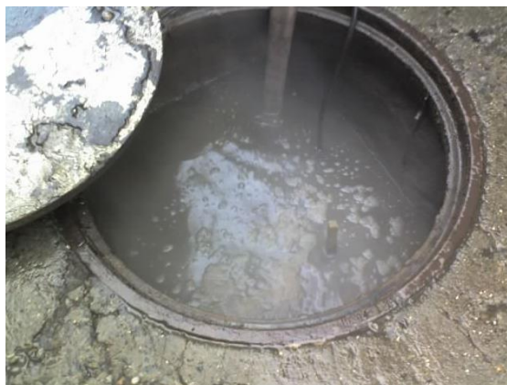
Flooded Manhole
