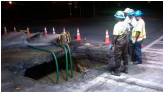
DeKalb County crews work to repair water main break
