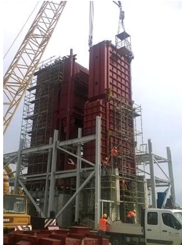
Boiler erection – Economizer lift
