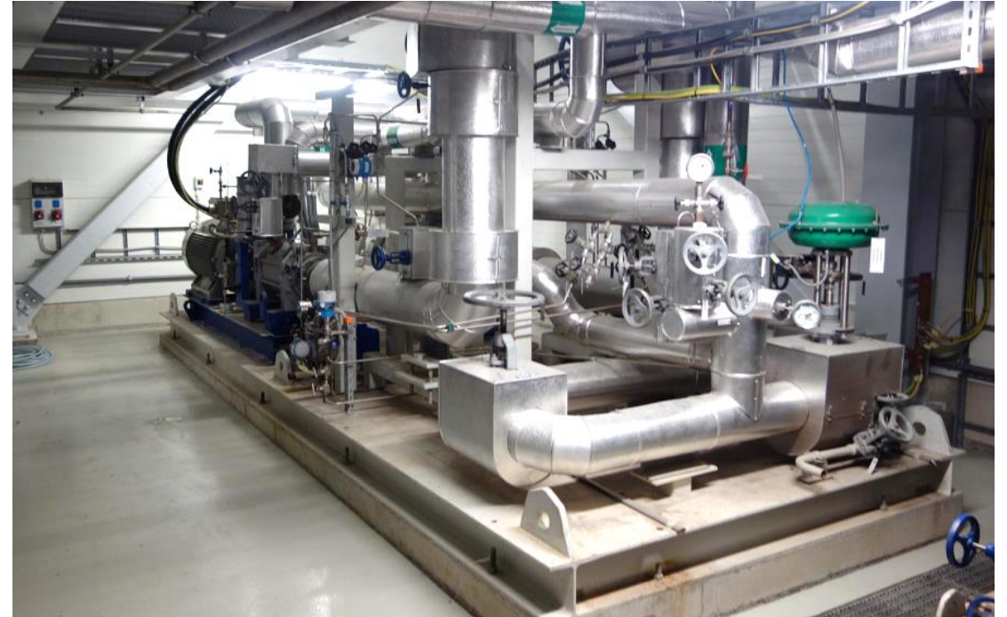
Feed water pump module in operation
