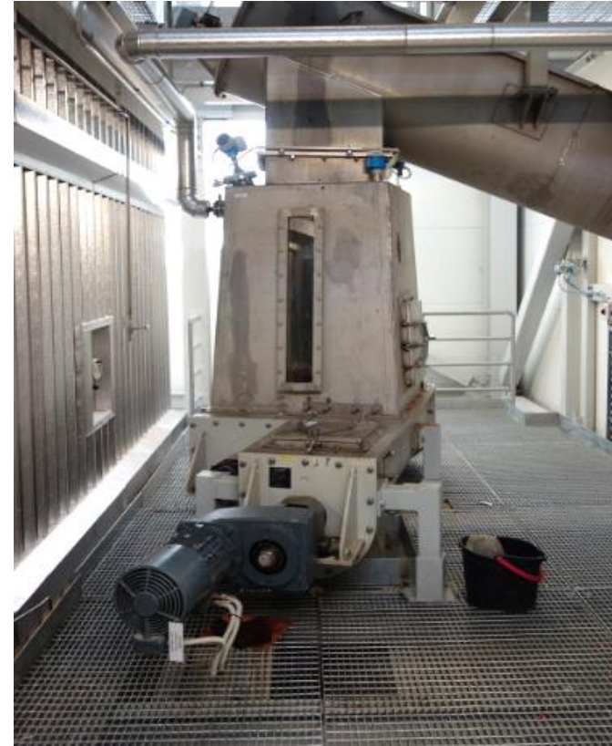
Boiler fuel feeding balancing bin - Fuel feeding is the key for efficient combustion and emission control
