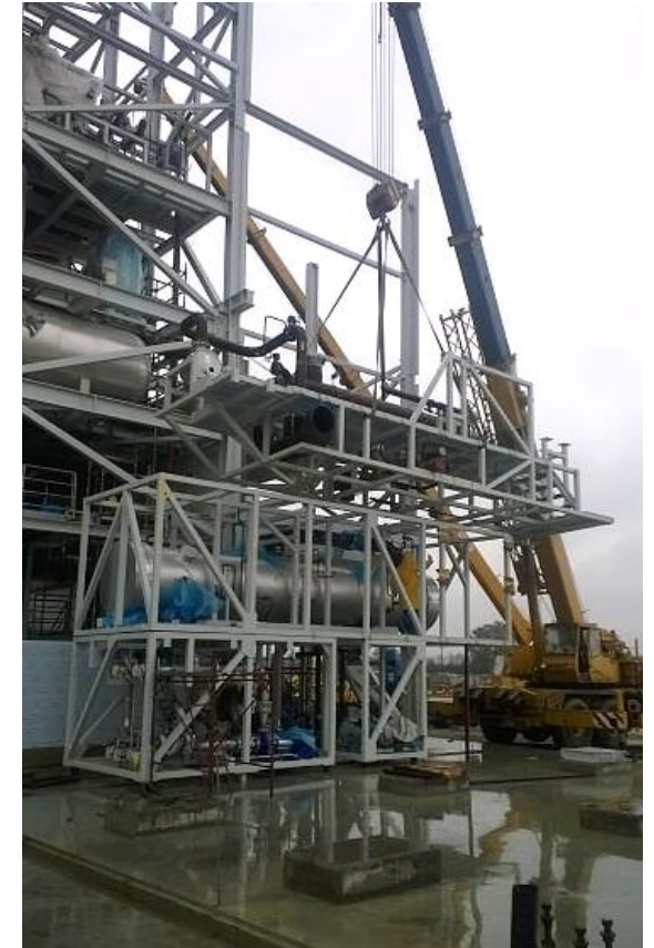
Lifting of the reduction valve module. The heat exchanger module tower combines five process modules with an integral stair tower for turbine hall
