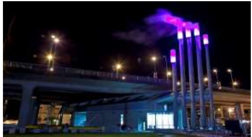
False Creek Energy Centre, Vancouver, BC
