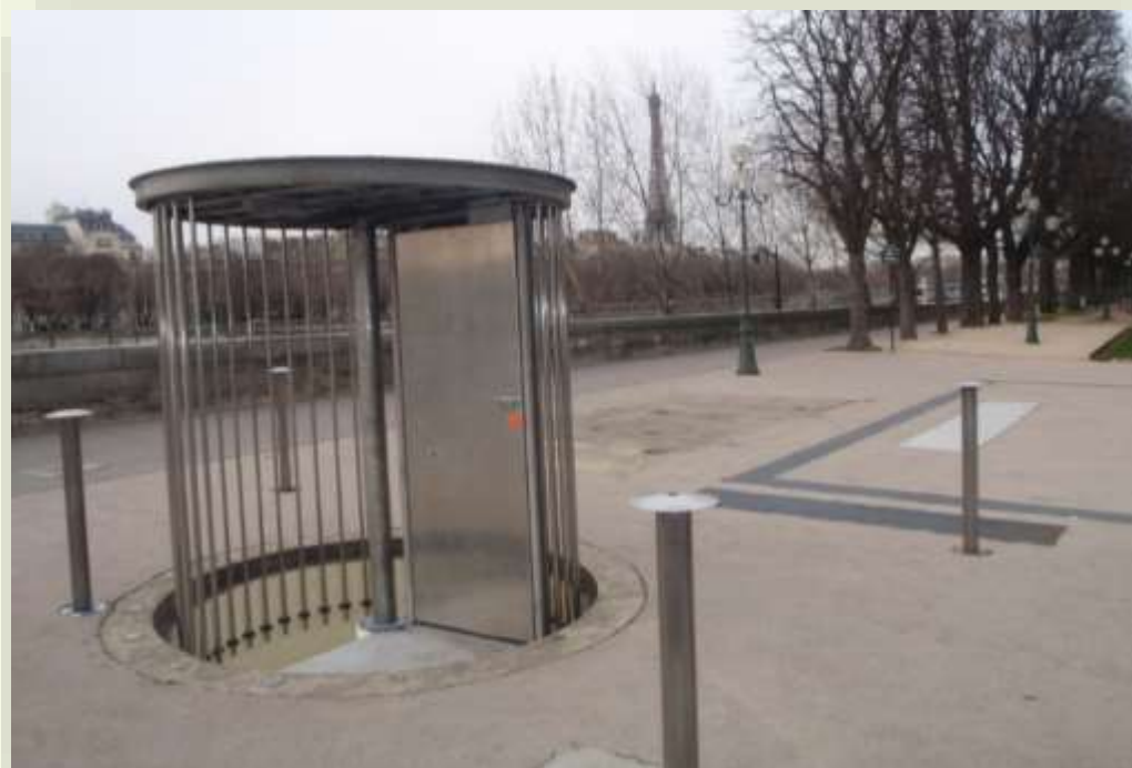
Entrance to Chilled Water Plant in Paris
