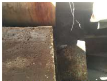
Rusted and Broken Anchor Plate on 6" 70S
