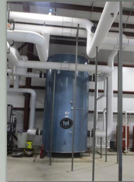
**Storage allows 5 mmBtu/hr boiler to meet higher demands from system**
