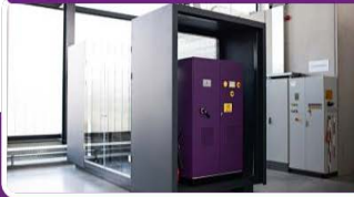
200 kW/200 kWh Li-Ion Battery
