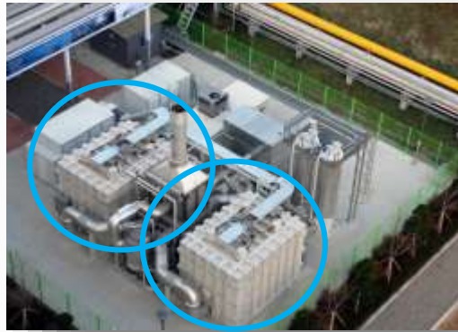
Two modules are used for a 2.8 MW power plant
