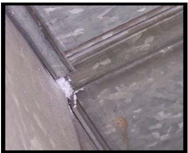
Doesn't coat the duct interior. Accumulates solely around the leaks.
