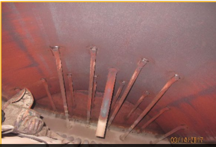
No wastage or weld cracks on diagonal stays
