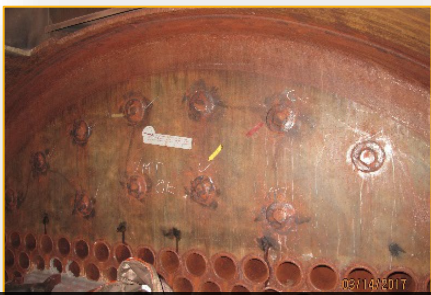
External stay welds tested
