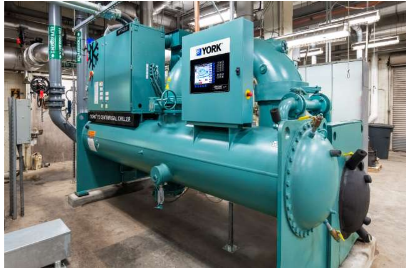
Magnetic bearing chiller installed in West Pickle Research Center mechanical room
