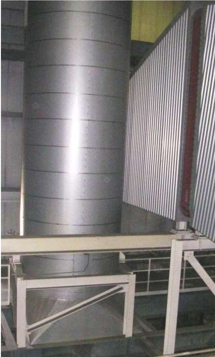
Duct cross connection
