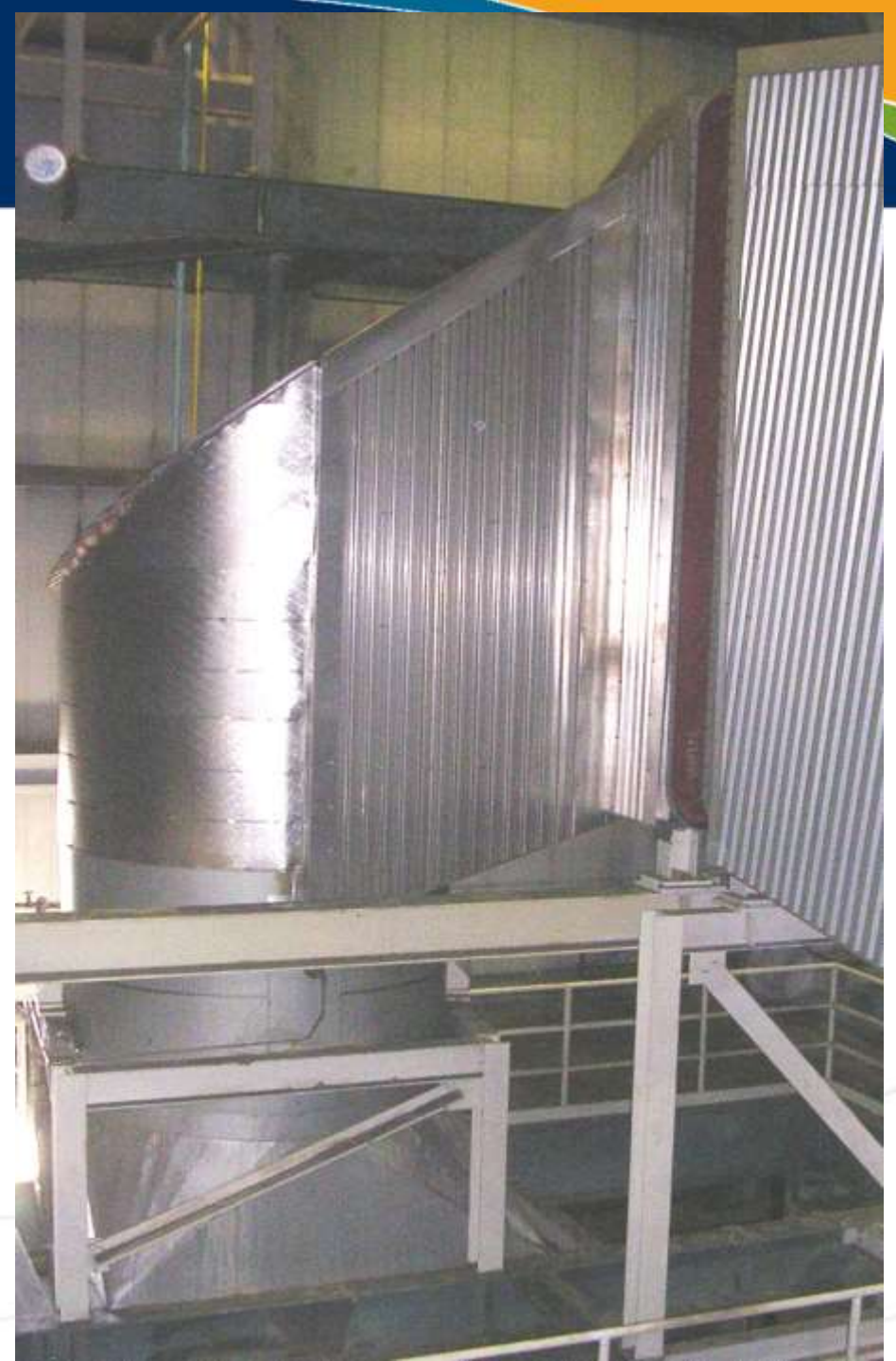
Duct cross connection
