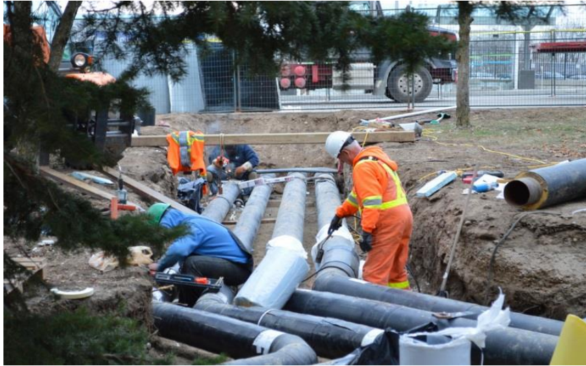
Image: Installing pipes as part of downtown Guelph, Ontario's heating and cooling system. Credit: Mike1024.
