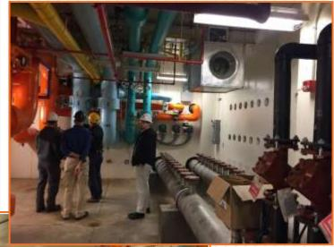
Well Field Headers entering basement of plant; note spare risers for future well headers. Basement allows for easy access.
