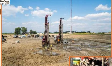
Installation of the Geothermal Well Field: 320 wells at 365 feet deep, 6" dia.
