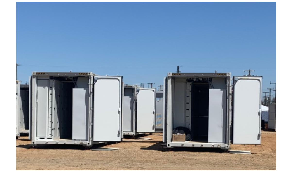
Battery modules were shipped within containers that were outfitted with battery management systems, lighting, fire detection, and fire suppression. The modules were factory wired to a DC combining disconnect. The battery containers were picked from delivery trucks and placed onto foundations.
