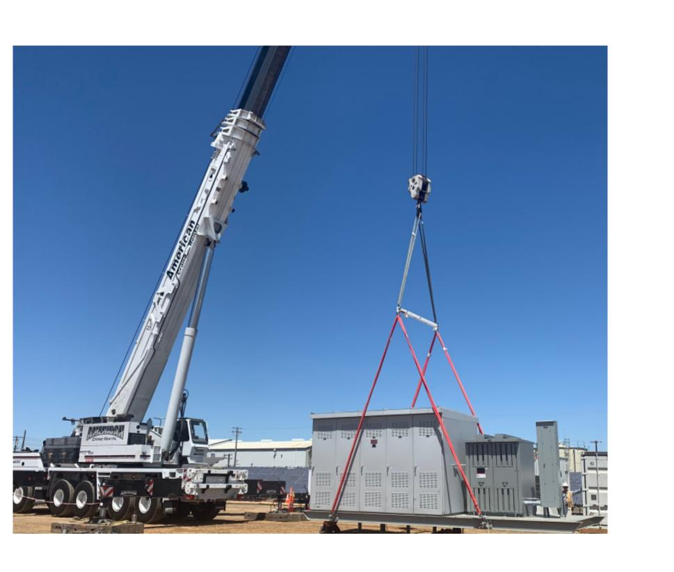
The remainder of the equipment was shipped to a skid integrator to mount and wire the equipment that was on the skid. The completed skid was shipped to the site, picked, and placed on the foundation system. The battery containers were then connected to the PCS skid and the PCS skid connected to a local distribution network.
