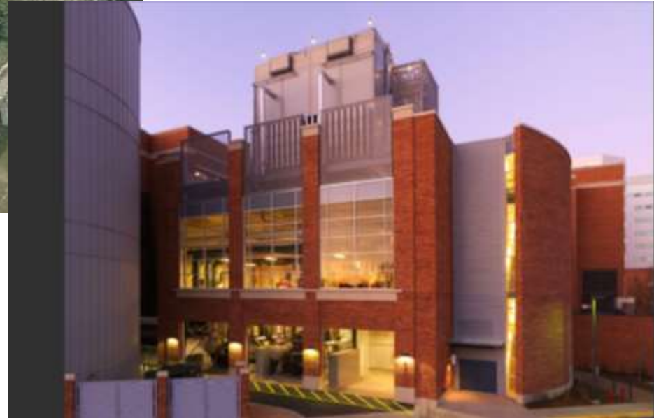
South Chiller Plant
