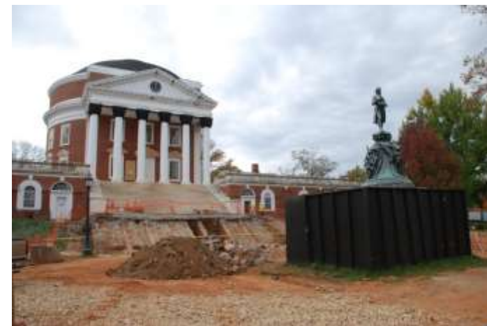
Jefferson' Rotunda – currently under renovation
