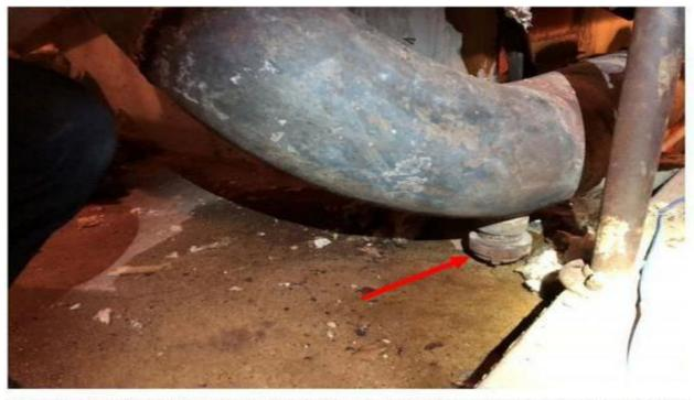
Figure 2: The location of the 2" drain and the failed cap. (All insulation has been removed as part of the investigation.)
