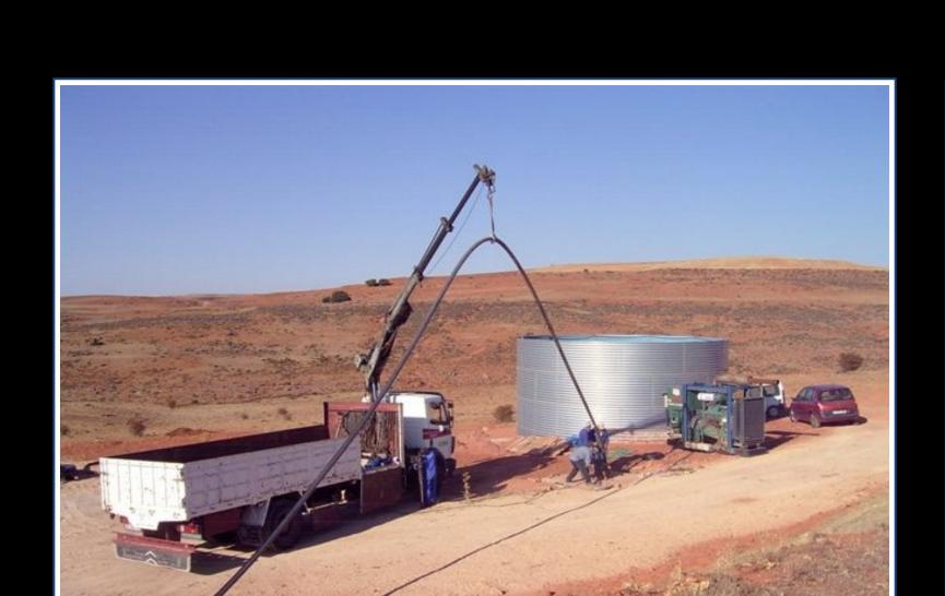
**NO CREEP:** BOREHOLE RIZER: Un supported while holding weight of pump, pipe, cable and water
