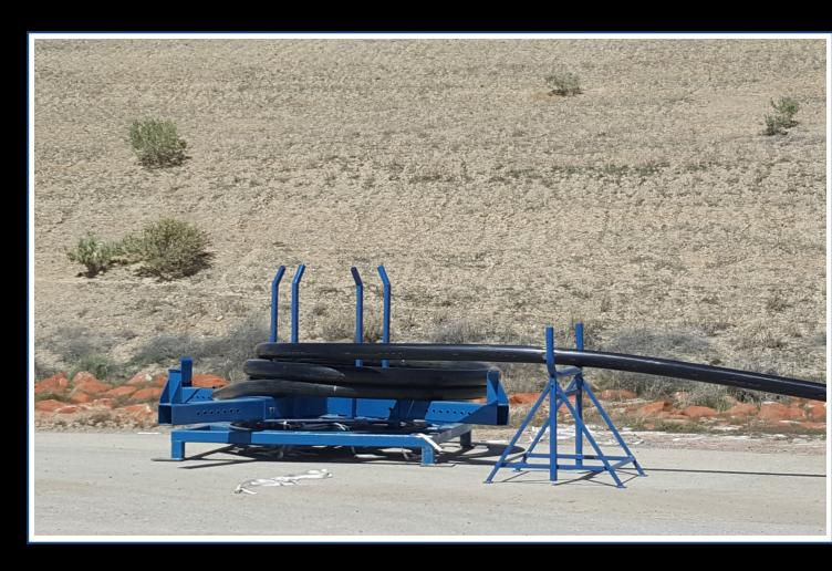
Coils Deployment: PE-Xa 8" DR11 3000ft in under 5 hours
