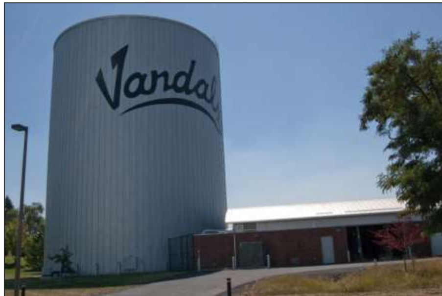
Figure 2. South campus chiller plant and cold TES
