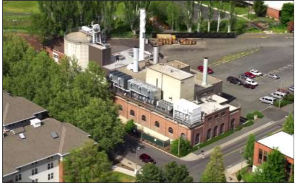
Figure 1. North campus energy plant
