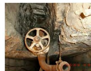
⑥ 7+36 TO 7+45 - ROOF WITH LARGE OPENING WITH VALVE AND BAR EXPOSED AND SPALLING
