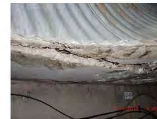
③ 7+20 - LARGE DELAMINATION ON ROOF SLAB AROUND PIPE
