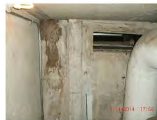
① 6+21 - EAST WALL LEAK AT CONSTRUCTION JOINT. GRATING DETACHED FROM OPENING
