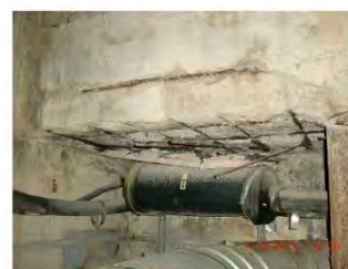
⑤ 7+30 - SEVERE ROOF SPALL
