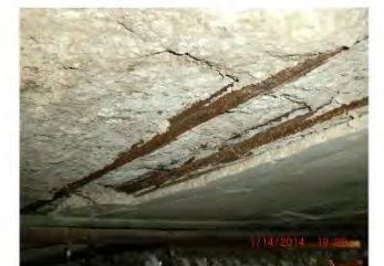
④ 7+25 - LARGE ROOF SPALL
