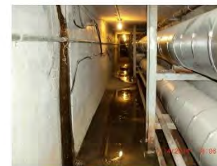
② 6+42 - CONDUIT LEAKING WATER INTO TUNNEL
