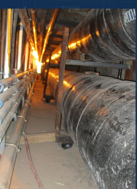
DIRECT BURIED STEAM LINES IN EXISTING RIVERSIDE VAULT. GROUT SOLID. SEE SHEET S1.01 AND S1.02 FOR MORE DETAILED INFORMATION.
