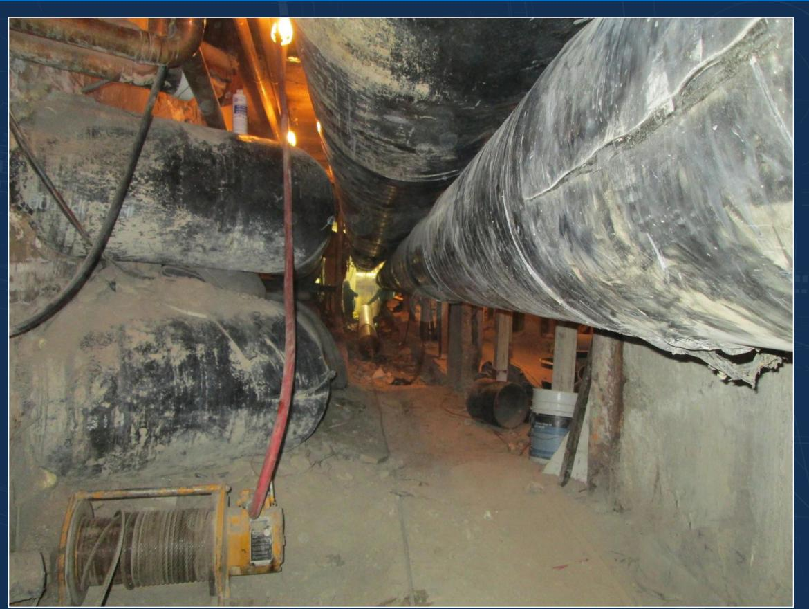
EXISTING 12" LF DIRECT BURIED STEAM RE-ROU TO BRIDGE ABUTMENT VAL
