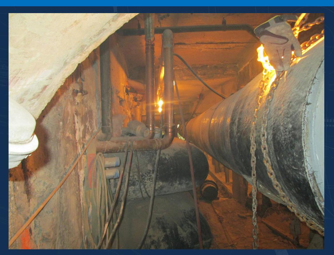
EXISTING 12" LF DIRECT BURIED STEAM RE-ROU TO BRIDGE ABUTMENT VAL
