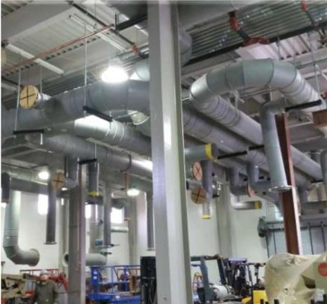
Most of the piping was fabricated at the factory to minimize the on site fusion welding.
