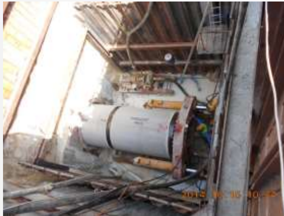
Driving the concrete pipes sleeves
