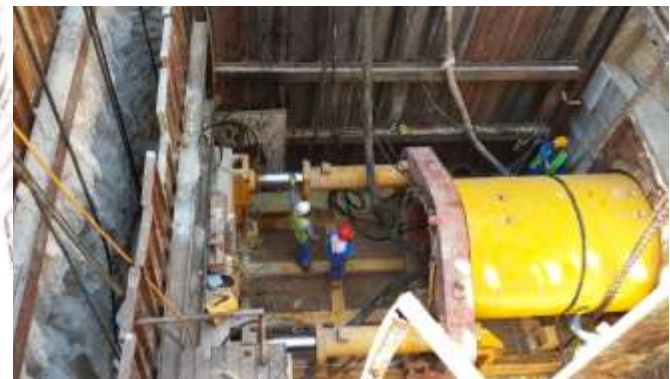
Installation of micro tunneling equipment at Driving Pit
