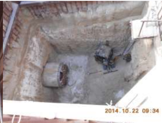
Completion of micro tunneling at Receiving Pit
