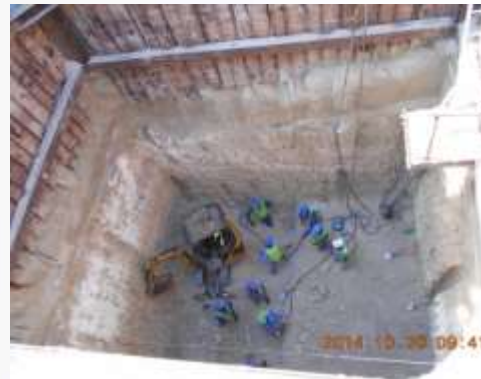
Excavating for Driving & Receiving Pits
