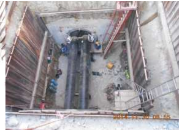
Installation of chilled water pipes inside the concrete sleeves
