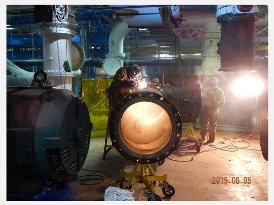
Field Erection of large bore piping
