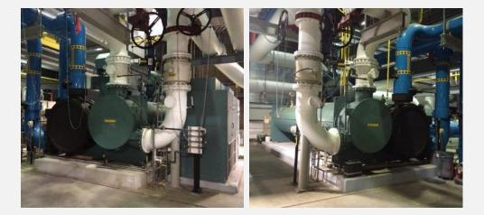
Installed two "half-size" chillers with pumps and piping.
