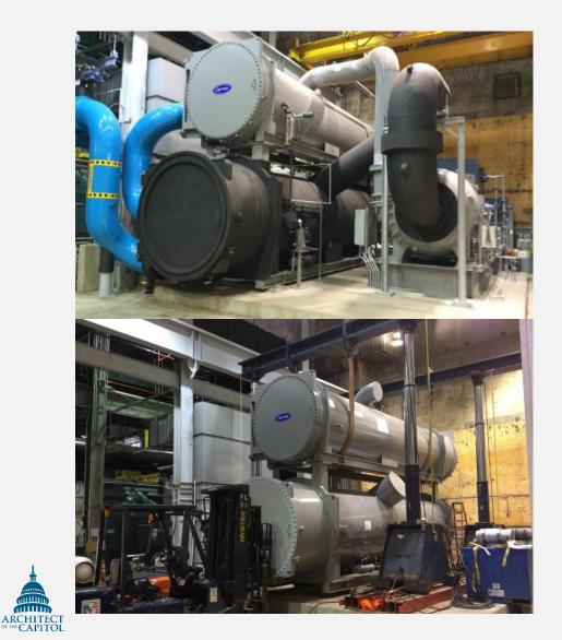
5,000 ton field-erected chillers were chosen for their high operational efficiency, and large cooling output for the required footprint
