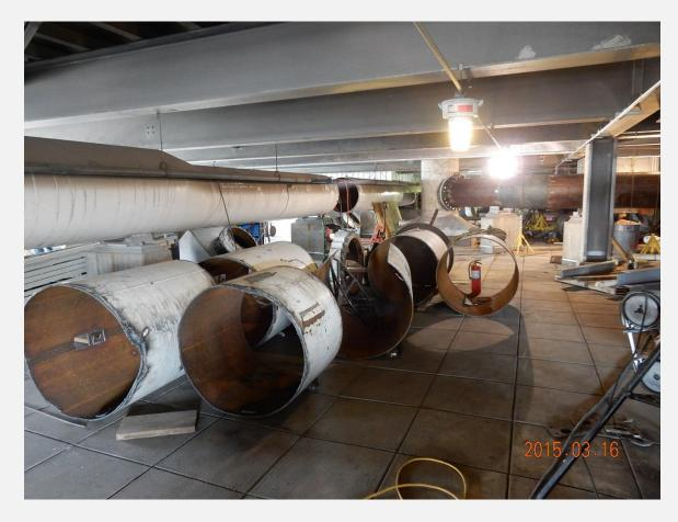
Installing new piping while leaving room to remove the old.
