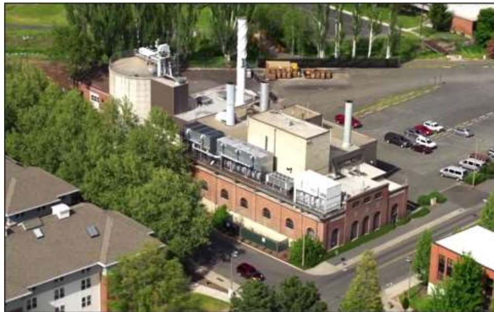
Figure 1: This is the UI district heating and cooling plant
