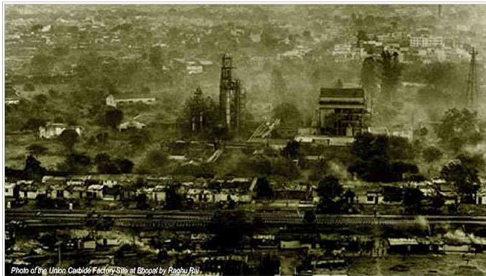
Photo of the Union Carbide Factory Site at Bhopal by Raghu Rai.
