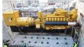
Engine gen. set in place at jobsite
