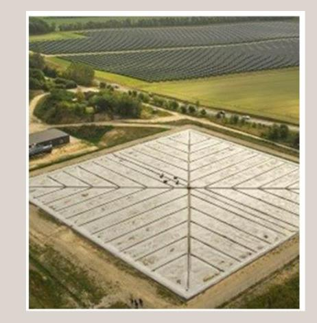
Dronninglund district heating utility in Denmark is the creator of one of the world's largest solar heating systems. A "reservoir" by 91x91 m / 300x300 ft water with a temperature in the 61,700 m<sup>3</sup>/ 16,2 mio gallons pool reaching app 90°C/ 195°F stores the solar energy from summer to winter.
