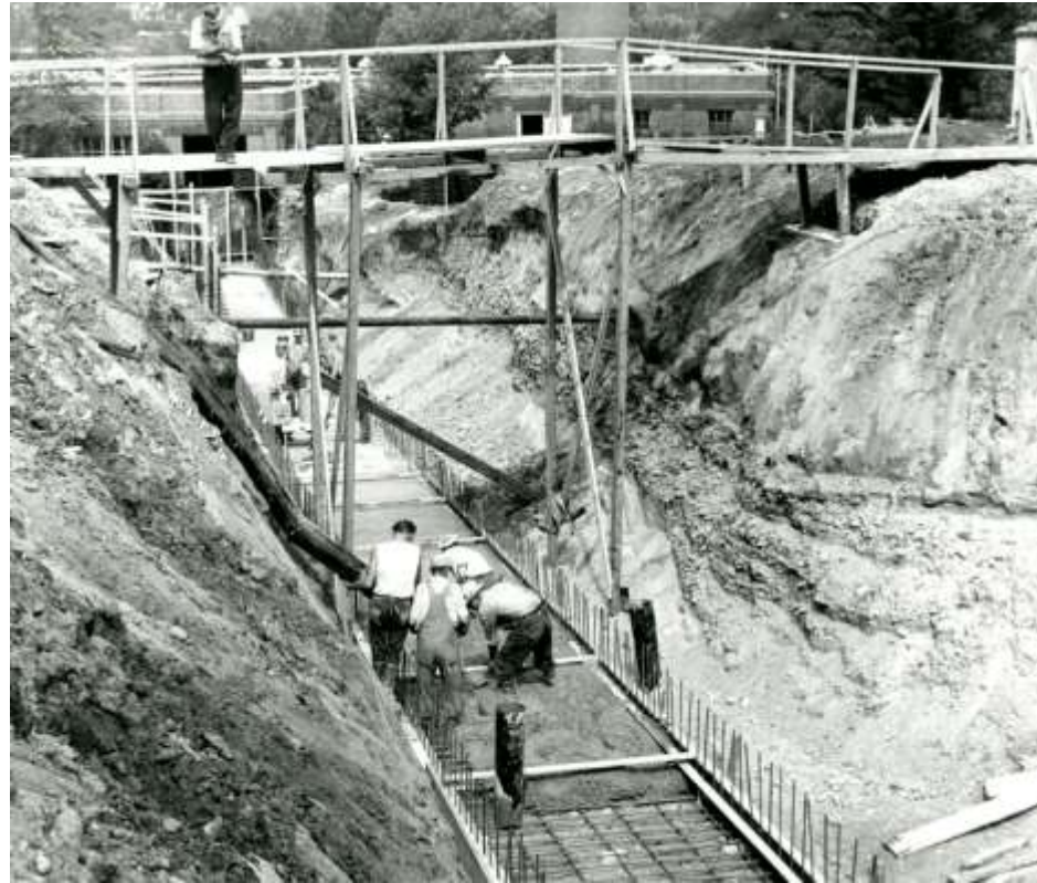
Expanding the steam tunnels
