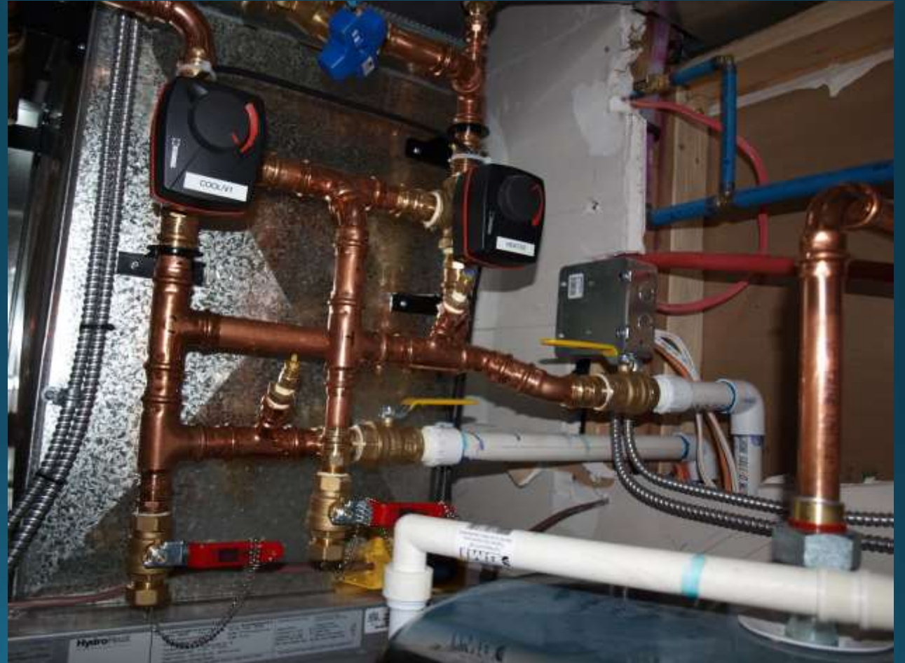
Detail of loop pipe connection to heat pump with 3-way valves for switching between heating and cooling.
