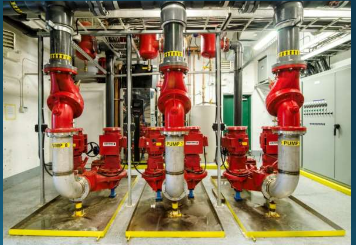
Double Head Bore Field Pumps for 100% Standby
