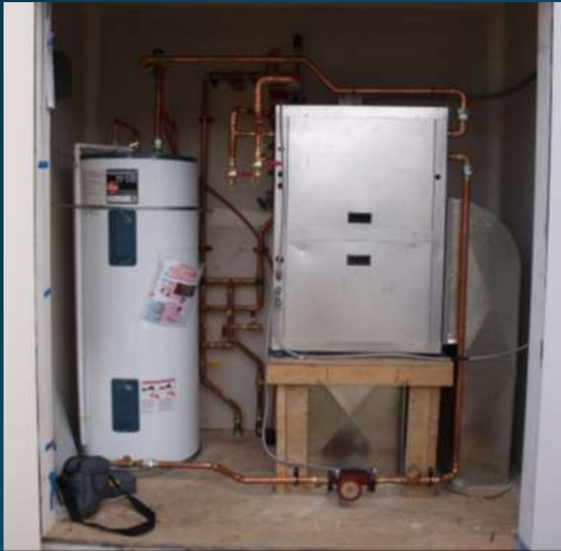
Heat pump and hot water tank accessed from outside.
