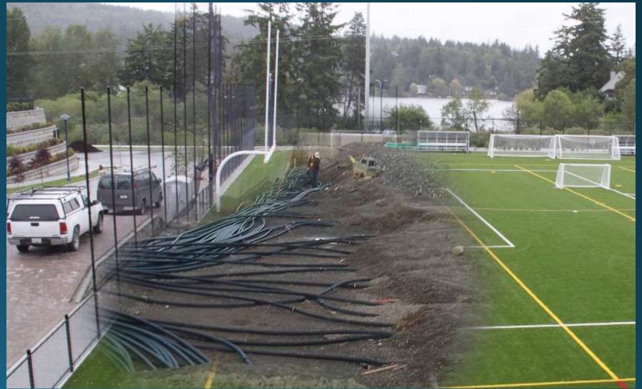
X-ray view of header pipes 6 feet below playing field
