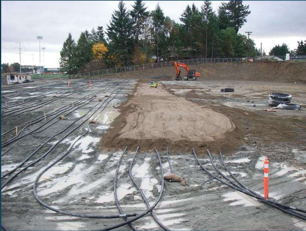
Header pipes in reverse return arrangement
