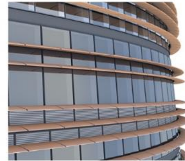
EXTERIOR FINS BLOCK DIRECT SOLAR IRRADIATION
