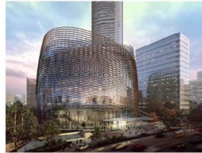
EXTERIOR FINS BLOCK DIRECT SOLAR IRRADIATION
