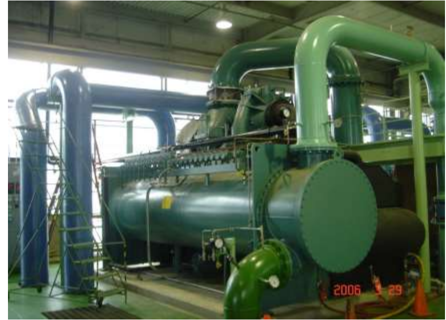
York YST Steam Drive Chillers, 600 Tons (2100 kW) to 2800 Tons (9800 kW)
