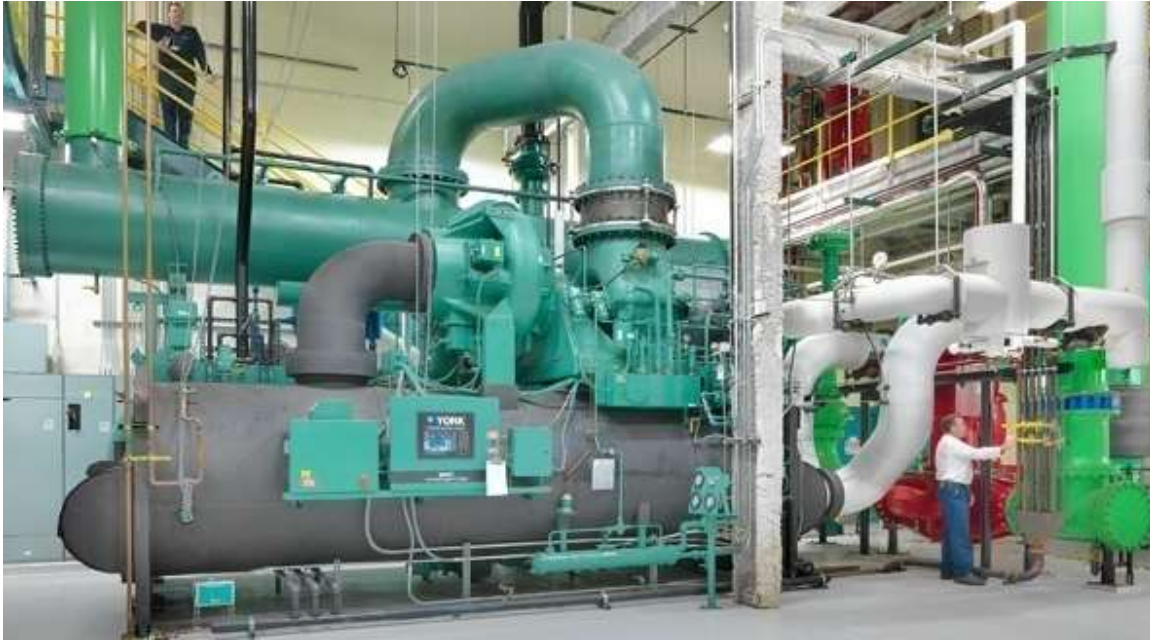
York YST Steam Drive Chillers, 600 Tons (2100 kW) to 2800 Tons (9800 kW)
