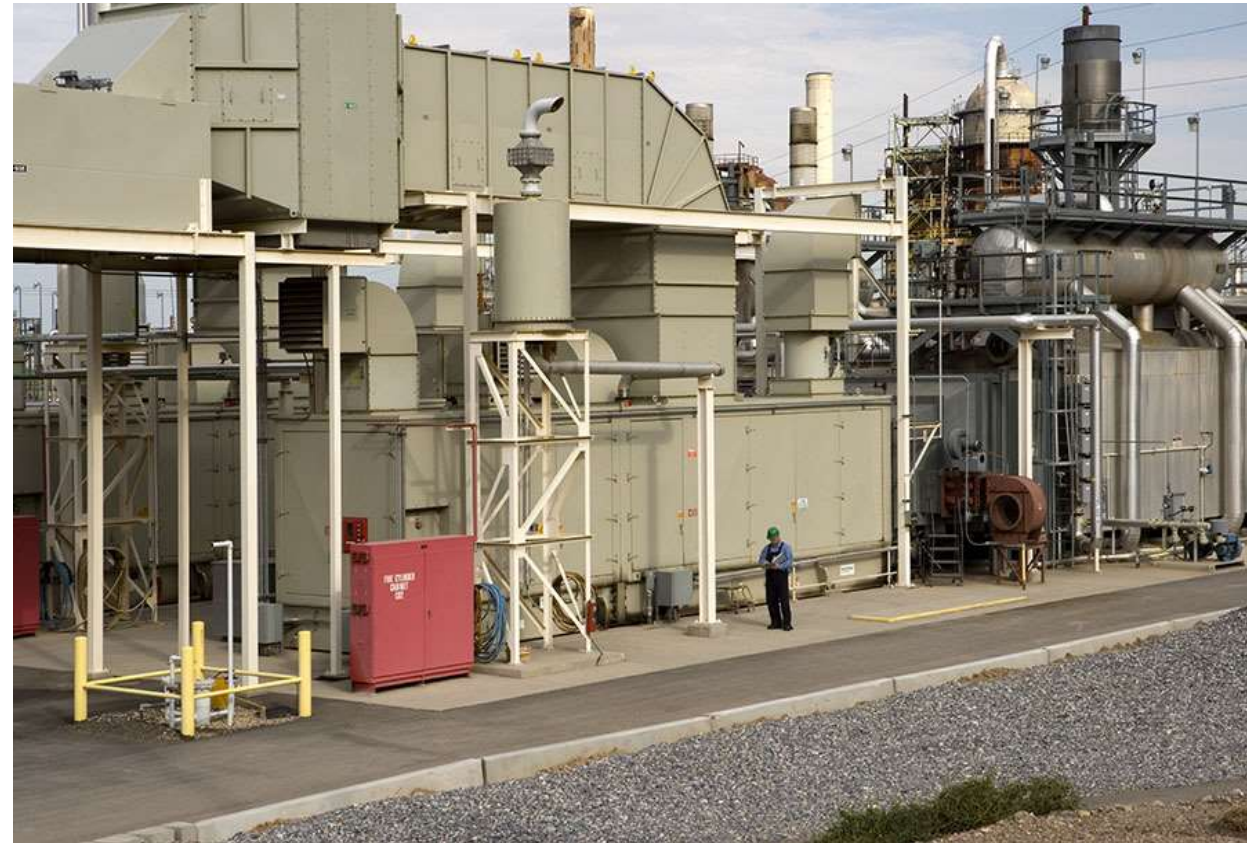
28 MWe Plant Using Hydrogen Refinery Off Gas
