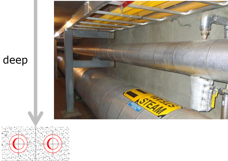
Steam – Concrete Duct
