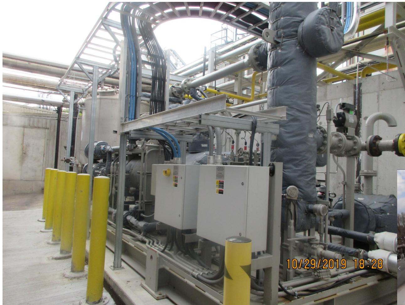
Fuel Gas Booster Compressor (FGBC)
